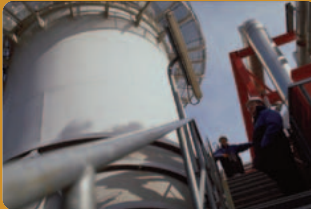
Sutton Bridge, EDF Energy's gas-fired power station
