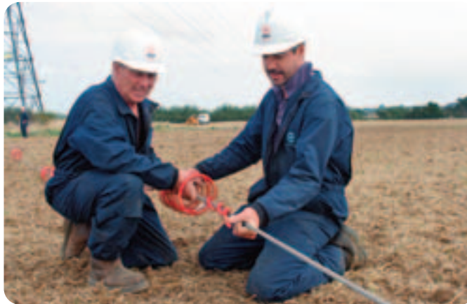
Employees fitting diverters to cables to protect swans
